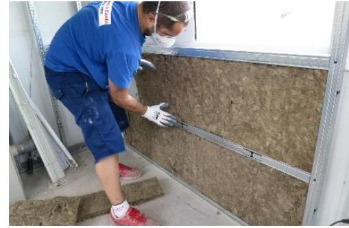
Thermal insulation can be fitted prior to the TRIMSOUND installation.
