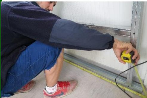
Wall being measured, in preparation for lining with plasterboard and TRIMSOUND
