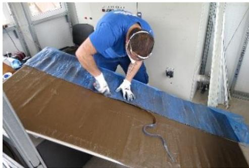
TRIMSOUND layer being lined to plasterboard. 600mm / 1200mm widths also available.
